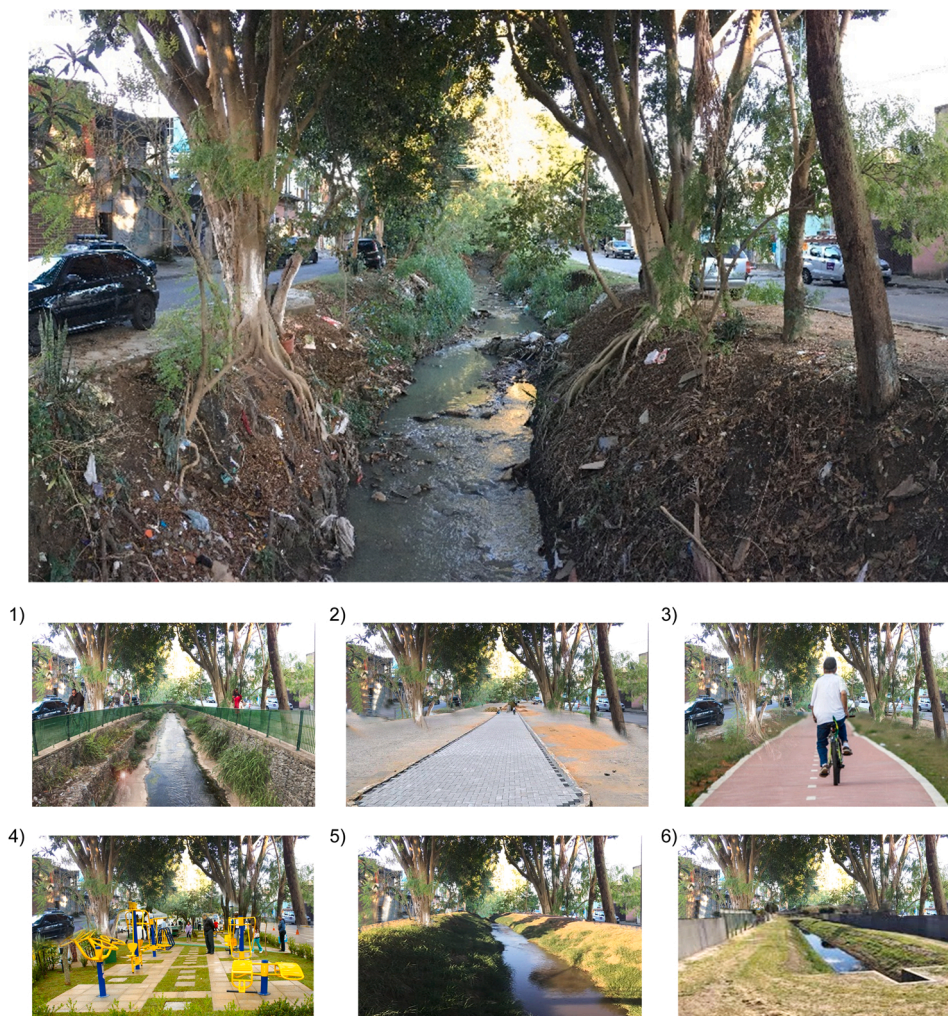
Fig. 6. Examples of digital simulations of river transformation scenarios discussed during Água Podre FGDs. Top: current (pre-intervention) situation; 1) surfacing stream with gabions and railing (as implemented in Sapé); 2) culverted stream with walkway; 3) culverted stream with cycling lane; 4) culverted stream with exercise equipment; 5) renaturalized river margins; 6) renaturalized river margins with railing.
